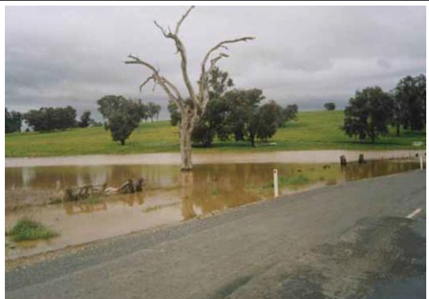
Plate C1.6 –Riverina Highway looking north east.
