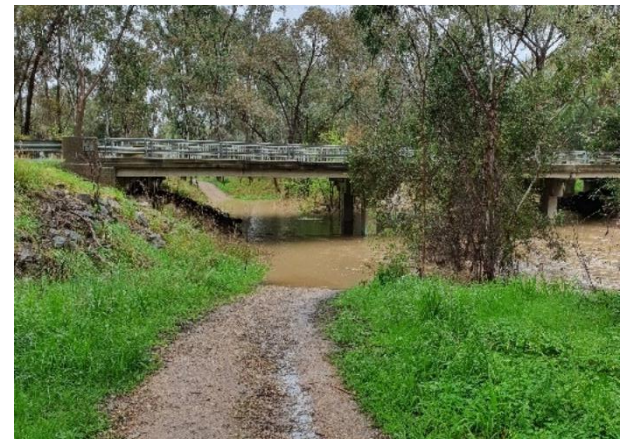
Plate C4.4 – Looking south east towards Thurgoona Drive crossing of Eight Mile Creek.
