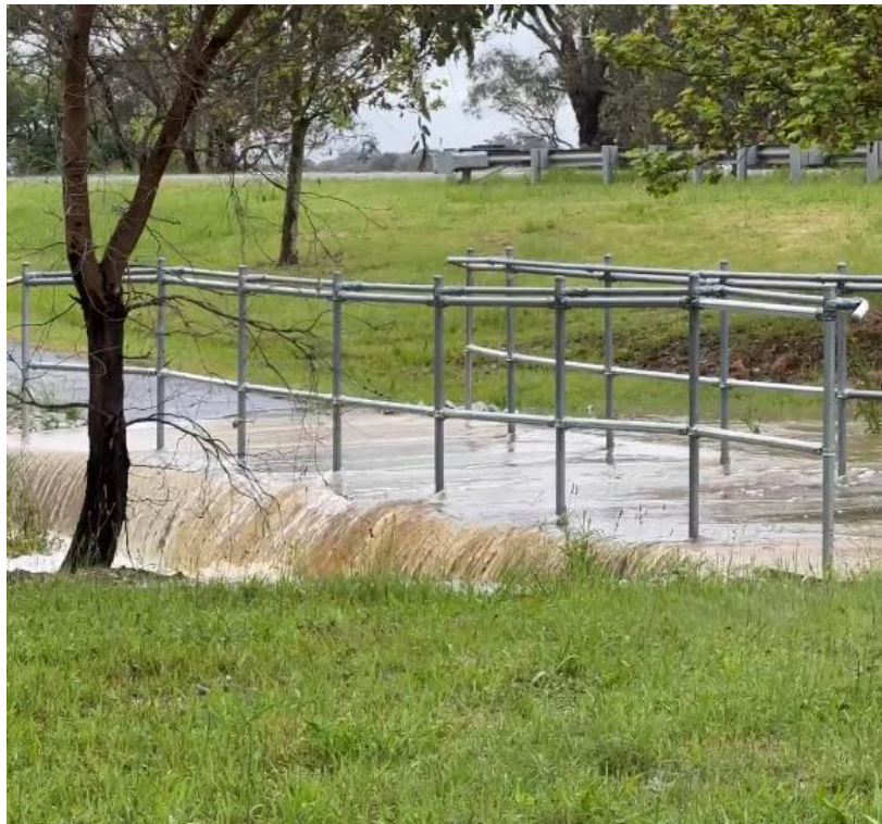
Plate C7.2 – Looking north-west from the southern side of the Riverina Highway, approximately 140m to the east of its intersection with Elizabeth Mitchell Drive.
